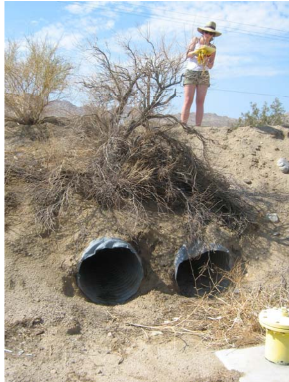
Figure 63. Pipe culverts on Highway 62 roughly 325 m west of Cascade Road.
