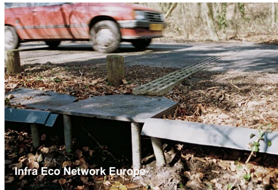
Figure 61. Amphibian tunnels allow light and moisture into the structure.
