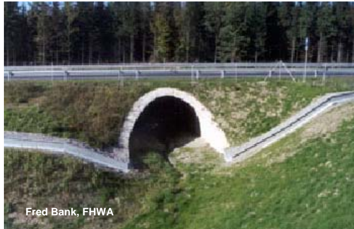
Figure 59. Arched culvert on German highway, with rail for amphibians and fence for larger animals.
