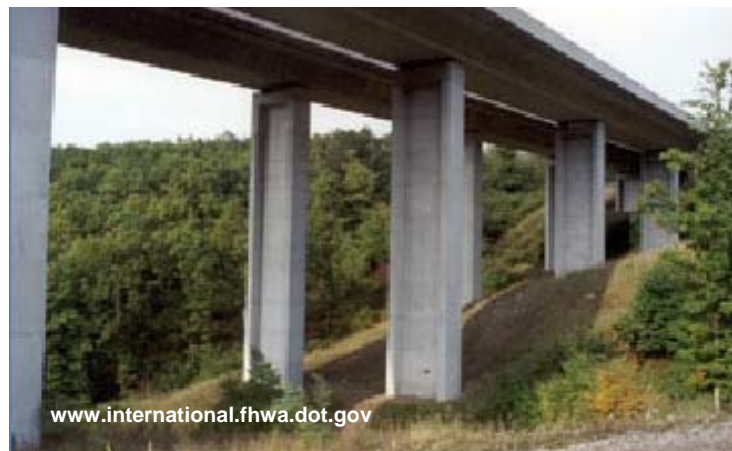
Figure 58. A viaduct in Slovenia built to accommodate wildlife, hydrology, and human connectivity.
